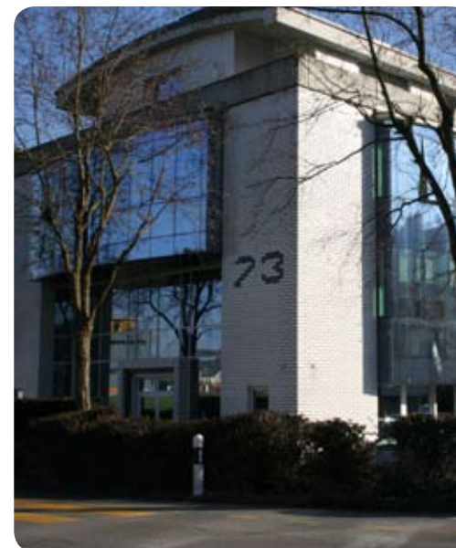
The headquarters of AUTOonline Schweiz AG in Pfäffikon.
